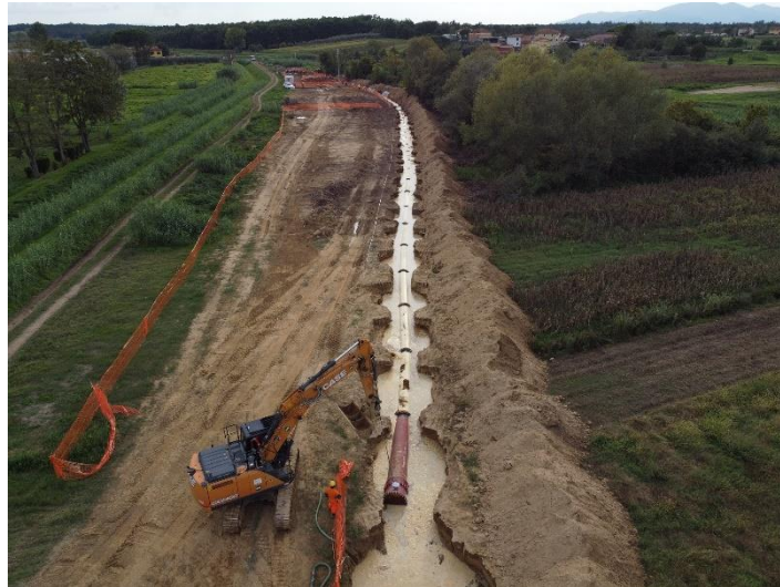
Figure 6. Aerial view of the pipe train being launched with flooded trench
